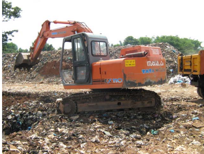
Removal of waste in segment B
