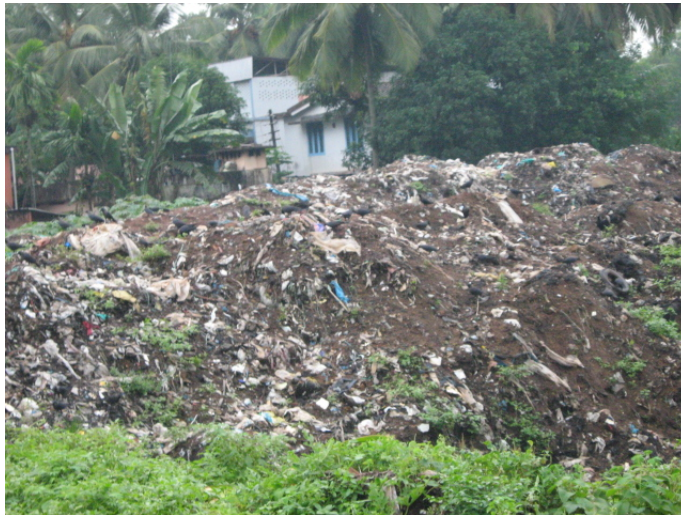
View of Excavated Material in segment B
